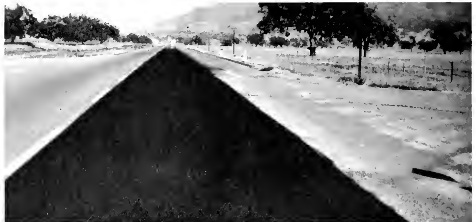
Completed slurry in right lane
